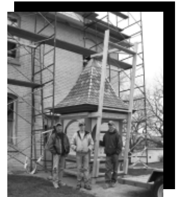
Lead Region Historic Trust Team preparing tower for hoisting
